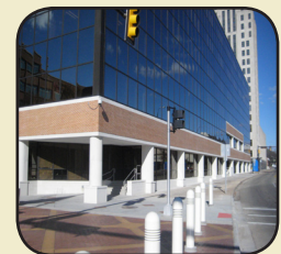
The facade renovation on 67 W. Michigan Avenue.
