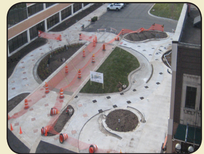
The Jackson Street Access Drive construction was completed in late 2010.
