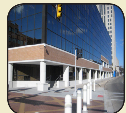
The facade renovation on 67 W. Michigan Avenue.
